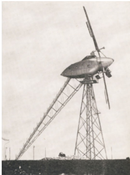
Soviet 100-KW wind turbine at Yalta 204
