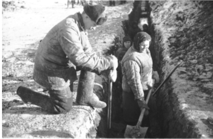
Construction of the natural gas pipeline to Kuybyshev, 1943 166
